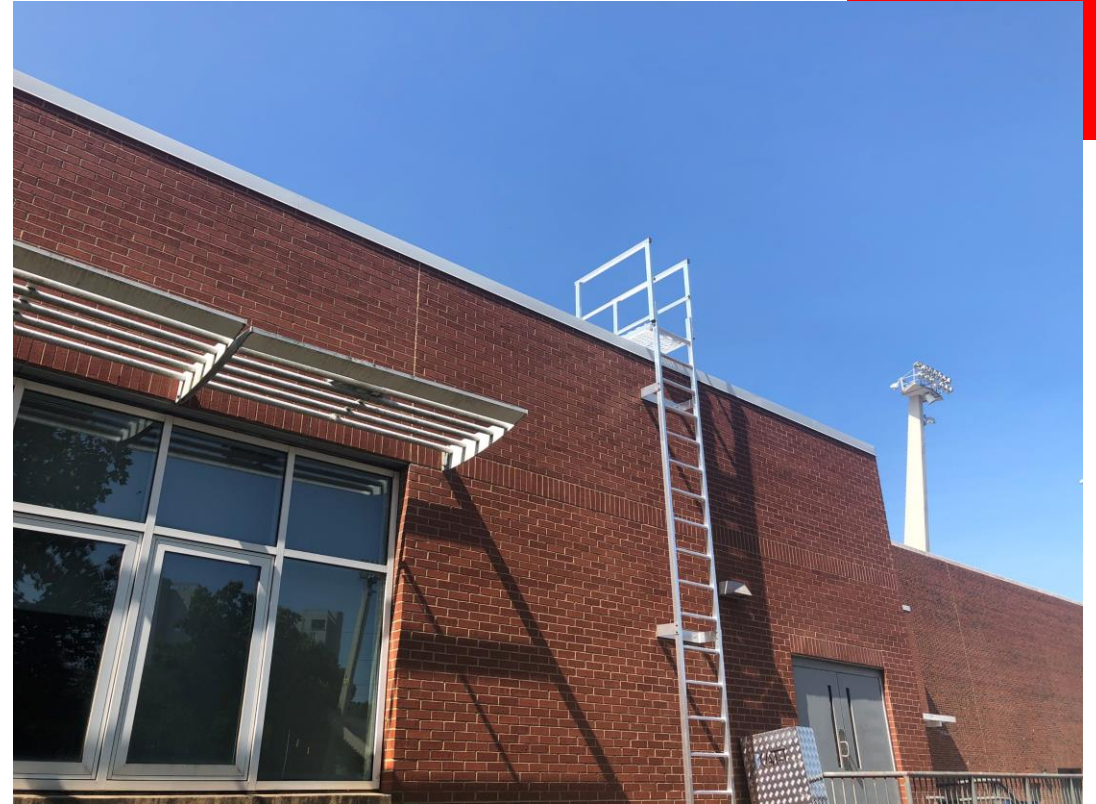
Roof Ladders Installed At Existing Buildings
